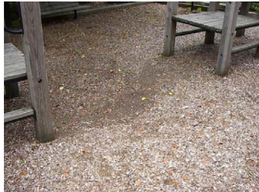
Worn Playground Surface
